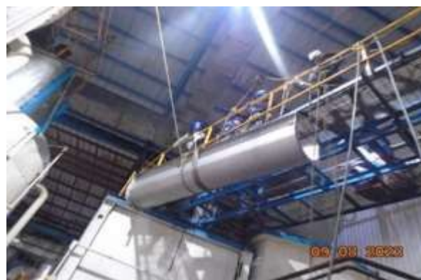
Figure 2. Leveling and alignment of the helical conveyor. Source: Prepared by the author.
