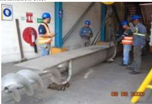
Figure 1. Helical conductor prepared for installation. Source: Author's own work.
