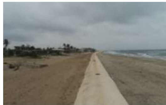
Figure 15. Figure showing the completion of beach protection works using geotextile fabric tubes, as well as sand filling on the beach in front of the geotextile fabric tubes.
