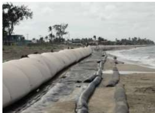
Figure 12. Geotextile fabric tubes on top of the anti-scour mat. Visualization of the project, its progress, and length at the construction site.
