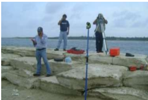
Figure 6. Figure showing the start of work with a topographic survey of the site where the work will be carried out in the community of Sánchez Magallanes.
