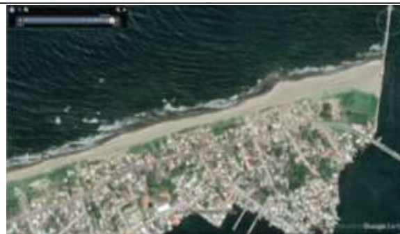
Figure 17. Figure showing the good physical condition of the beach protection and the material recovered from it in 2021, in the community of Sánchez Magallanes, Tabasco, Mexico.
