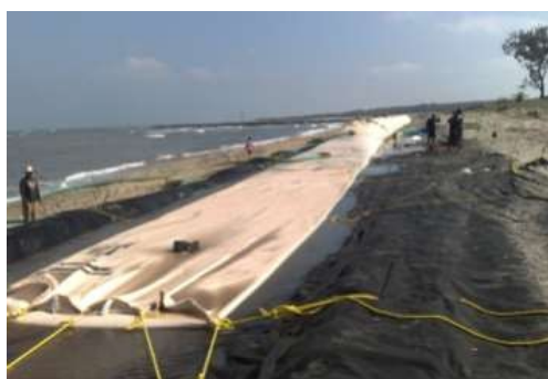
Figure 10. Figure showing the anti-scour mat already in place and the start of the installation of the geotextile tube to be filled with water and sand.
