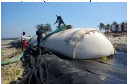
Figure 11. The laying and placement of the anti-scour mat and the filling of the geotextile fabric tube on top of the mat can be seen. The geotextile fabric tube is filled with water and sand using the 7.5 HP pump. The sand remains inside the tube, while the water flows out.
