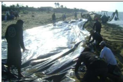
Figure 9. Placement of the anti-scour mat in the area and length where the geotextile tube will subsequently be placed.
