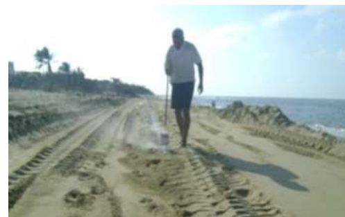
Figure 8. Figure showing the cleaning of the beach protection site, as well as the leveled ground and a person marking the line where the anti-scour mat and geotextile pipe will be placed.
