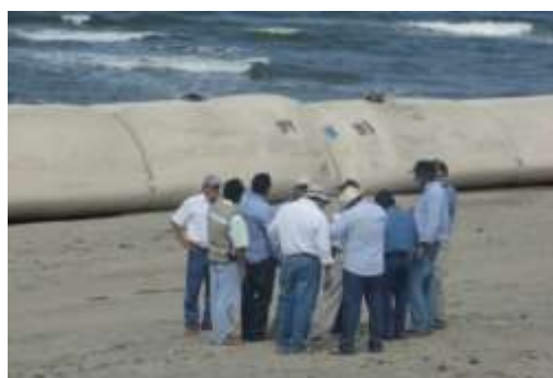
Figure 13. Meeting at the construction site between personnel from the Ministry of Communications and Transportation (SCT), the construction contractor, and supervisors to verify the beach construction work.
