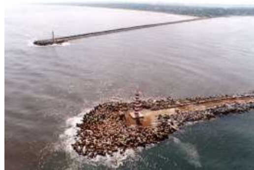
Figure 2. Example of breakwaters in the port of Coatzacoalcos, Veracruz. (Ramírez, 2009).
